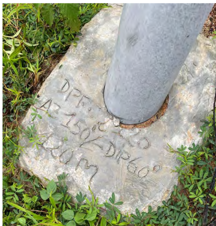
Figure 10.2 An Example of a Concrete Plinth Set Around PVC Casing at Souwa
